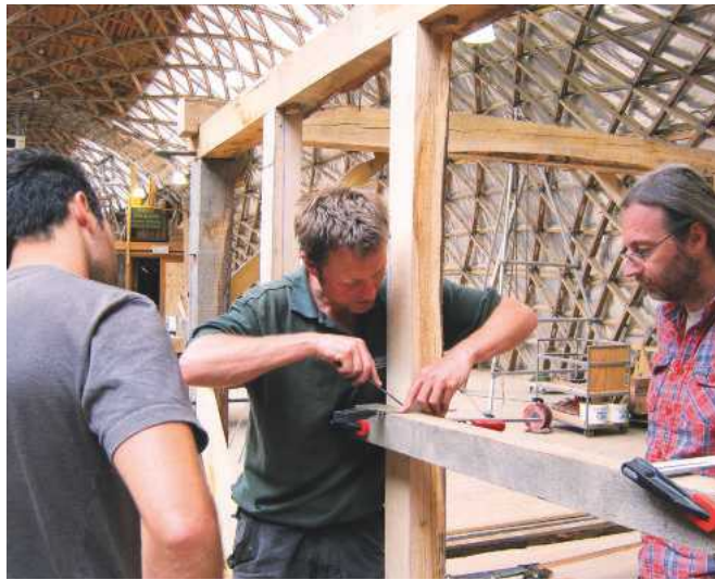
Timber framing in the modern Gridshell building
